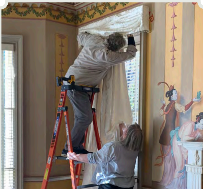
Bruce and Natalie Larson installing the dining room curtains.
