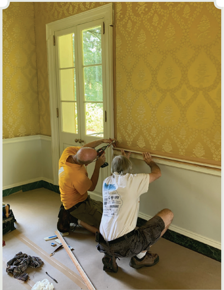
Keith Miller and Steve Tillander of Restoration Craftsmen installing trim
