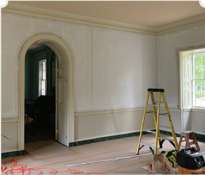
Batting installed on library walls
