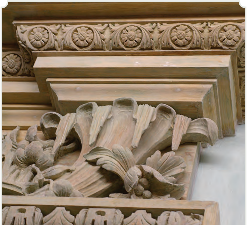
Detail of living room plasterwork, before restoration
