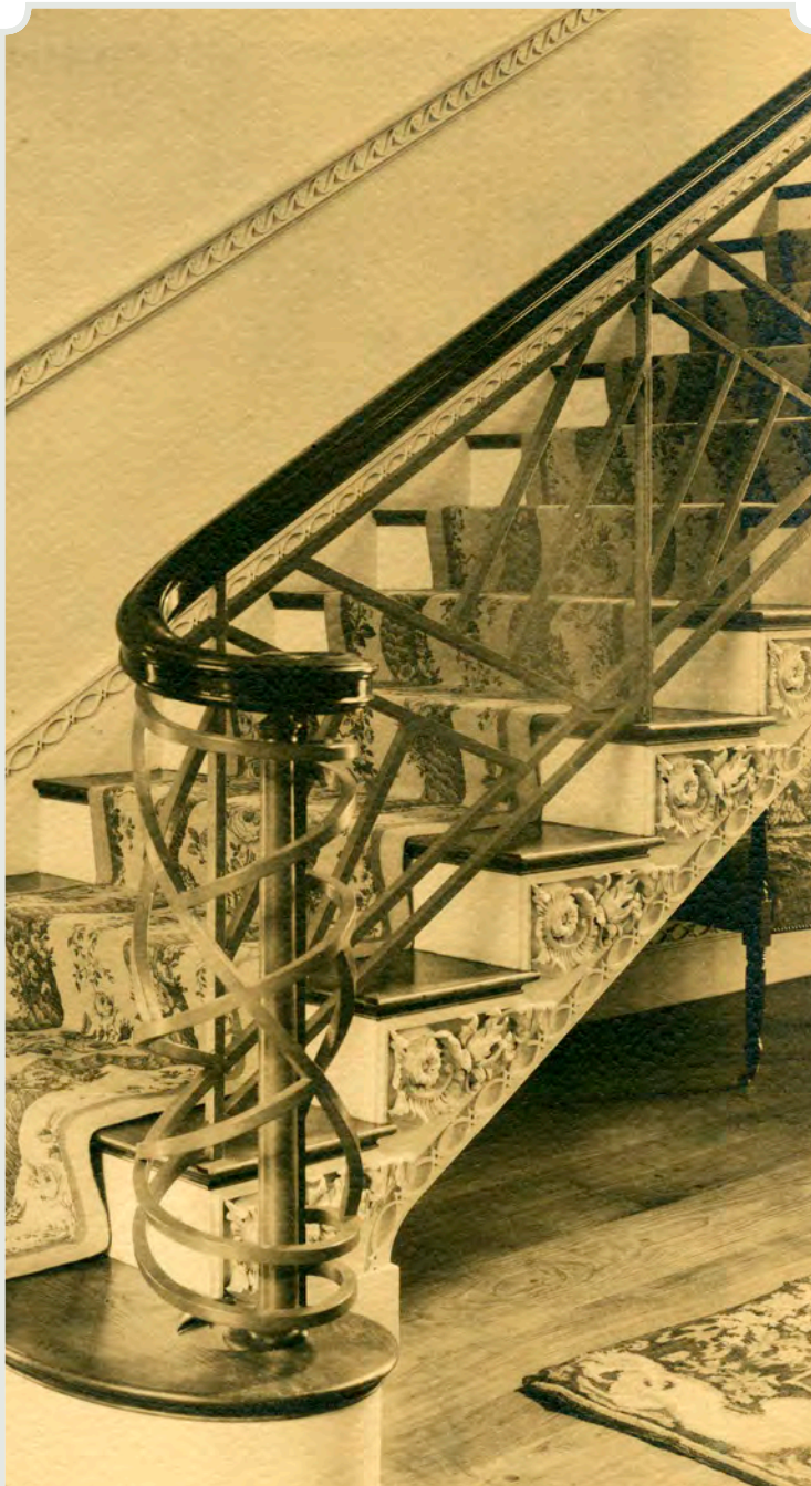
Staircase, May Patterson Goodrum House, 1931, Philip Trammell Shutze papers, MSS439, James G. Kenan Research Center at the Atlanta History Center
