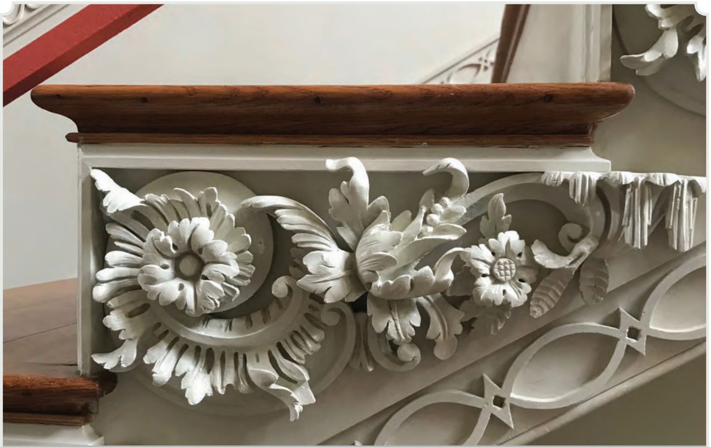
Detail of stair bracket, after restoration
