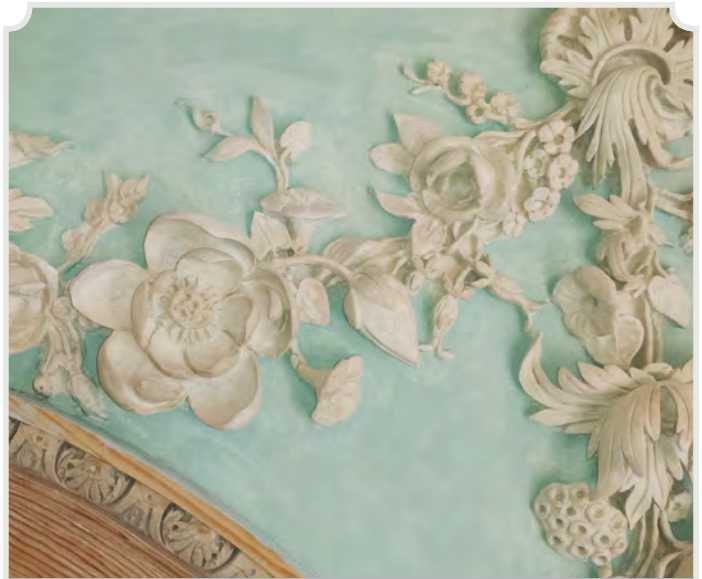
Detail of living room overdoor plasterwork, during restoration
