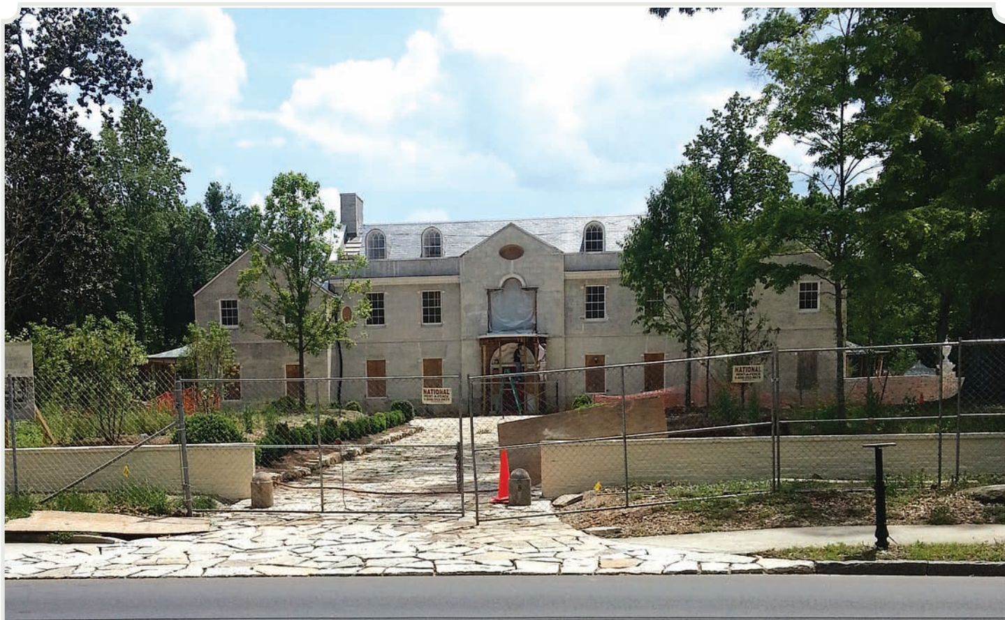
Granite spall drive apron at West Paces Ferry Road entrance.
