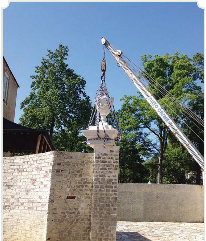
Cast decorative urn at service drive removed for evaluation and restoration.
