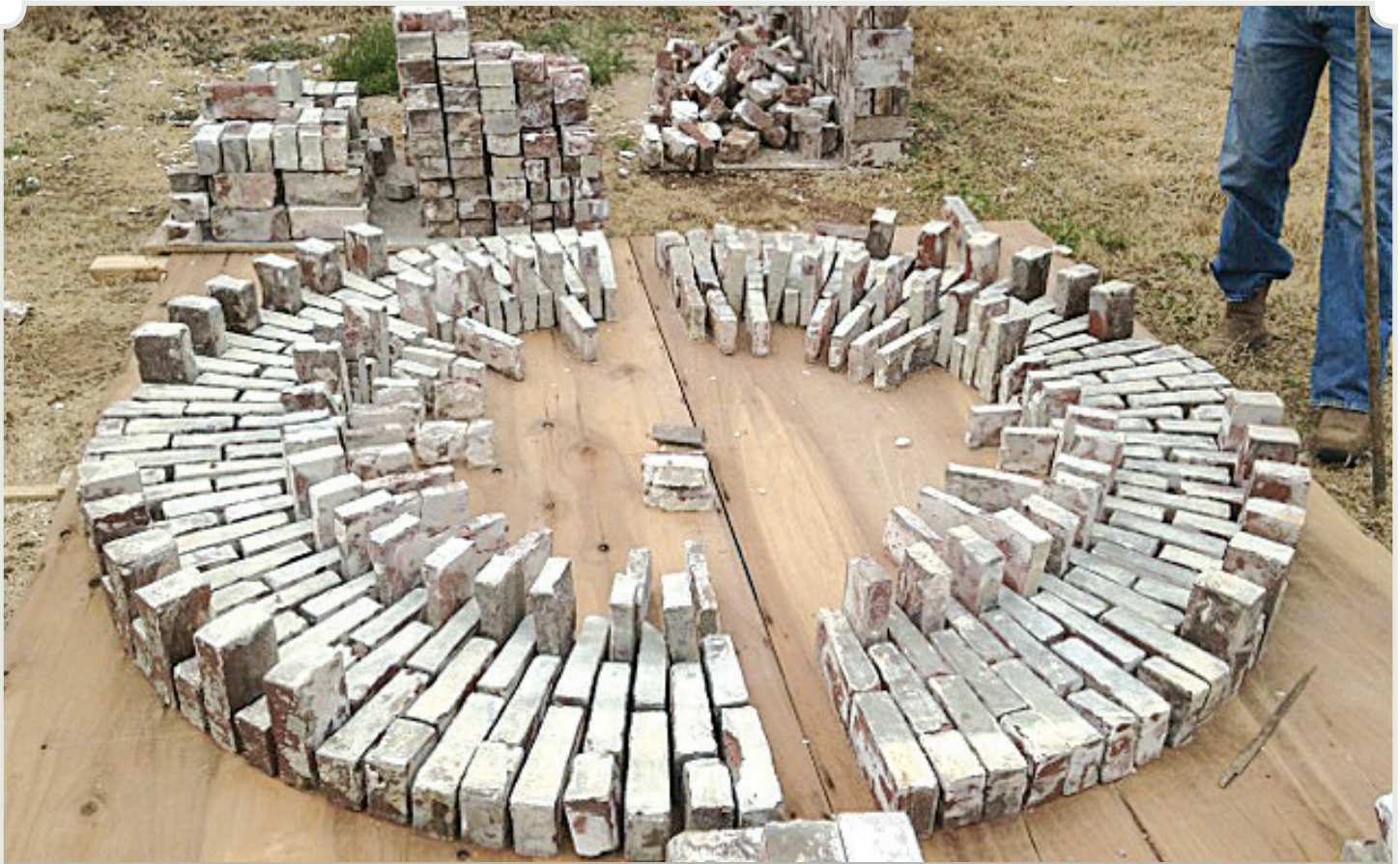
Individual bricks from arch at serpentine garden entrance dismantled and numbered in proper sequence.
